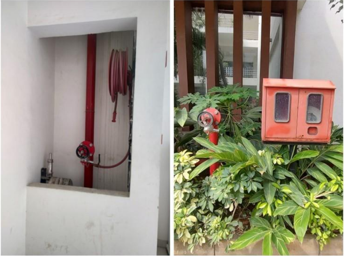
Figure 3-2: Fire hydrant system
