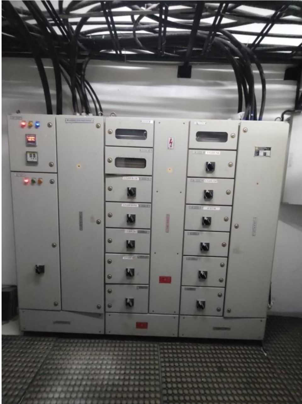
Figure 5-12: Electrical safety mats near electrical panel
