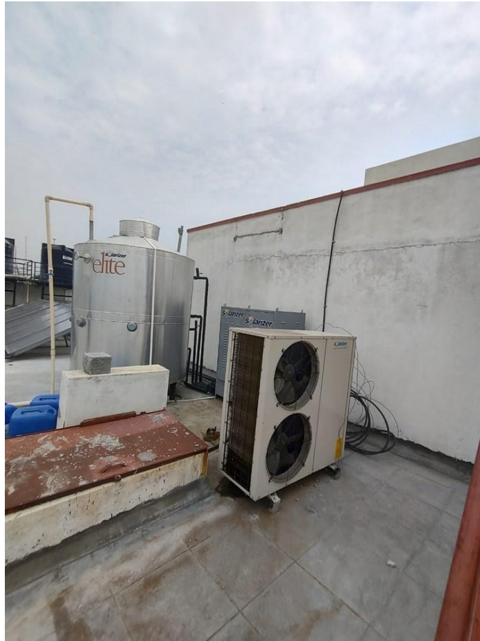
Figure 5-8: Integrated recirculation type -Hot water system
