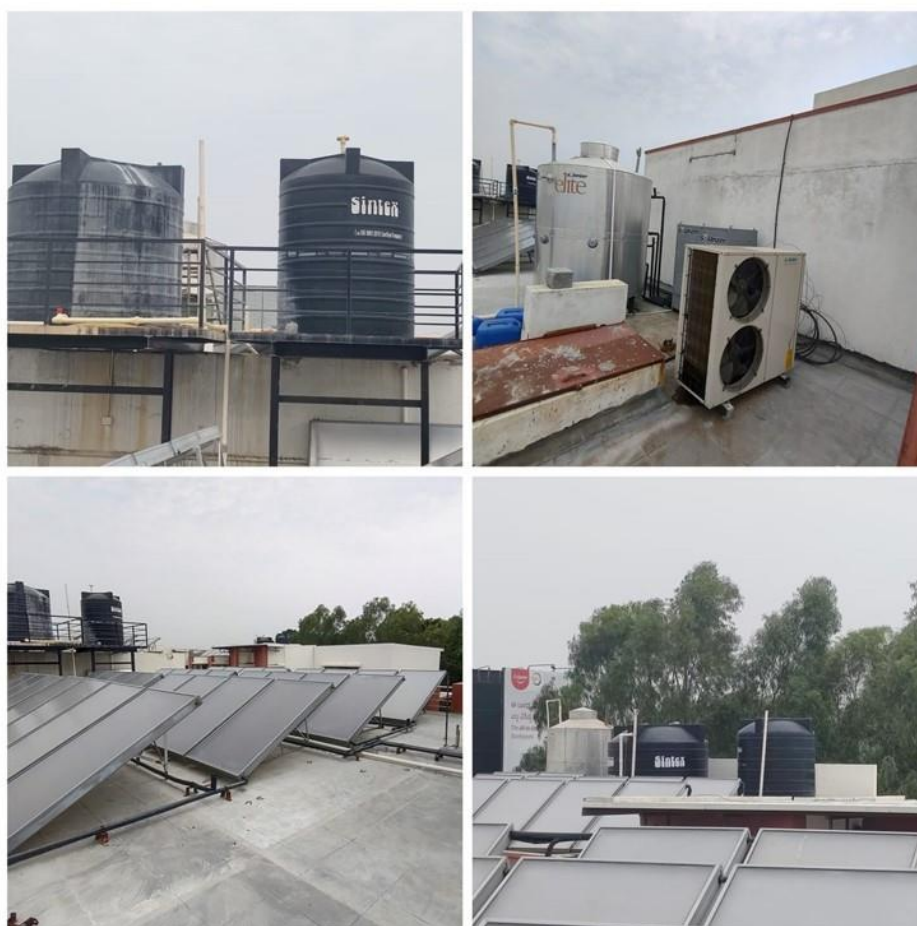
Figure 4-3: PVC Overhead tanks installed at the terrace
