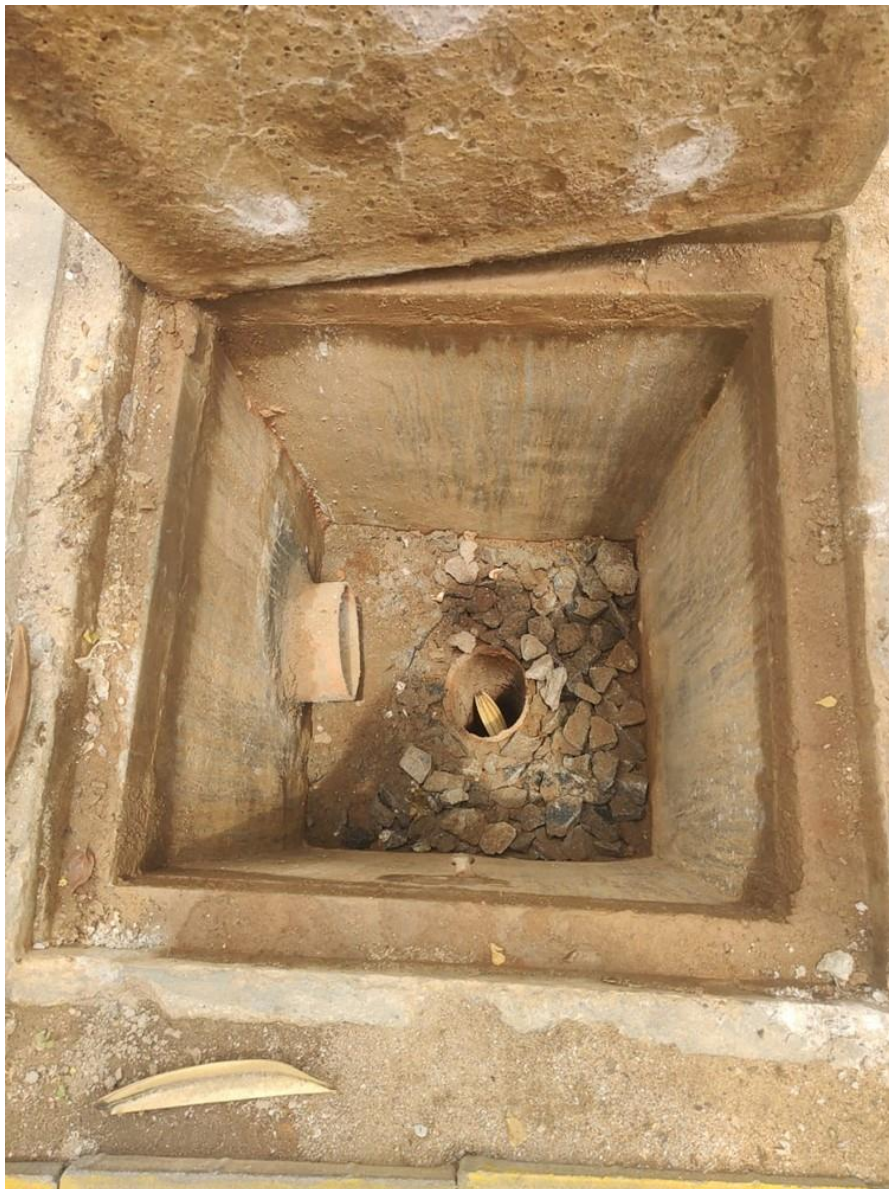
Figure 4-9: Ground water recharge pit
